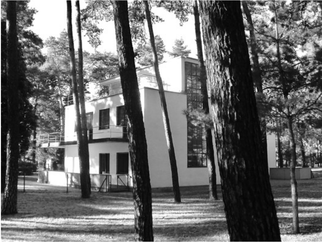
Figure 6. The Masters' Houses, Dessau. Designed by Walter Gropius in 1925 to house the Bauhaus professors.
